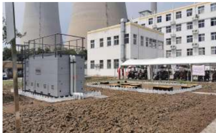
Water Treatment EPC Project
